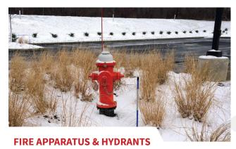
Stake fire apparatus and hydrants, utility boxes, gas meters, sewer vent pipes and other public safety hazards. Install adjacent to each fire hydrant, valve, standpipe or other apparatus. Blocking hydrants not only creates accessibility issues during an emergency but may also result in monetary fines.
