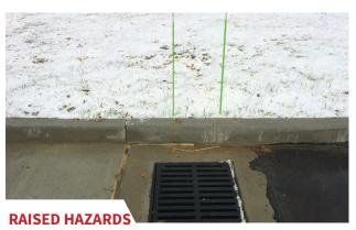
Stake catch basins, drainage areas, manholes covers or other areas that may catch a plow blade. Install on either side of the hazard, or if it is in the center of a lot, place stakes on leading and back edges of the hazards in a noticeable location along curb lines across from the basin. Drains should be kept clear to prevent ice jamming and clogging.
